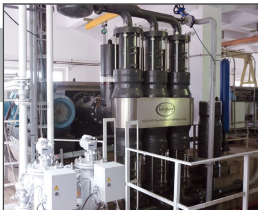
FELUWA MULTISAFE® double hose-diaphragm process pump. One triplex unit (out of three) in a dense ash pipeline disposal system. Q = 150 \text{ m}^3/\text{h} each p = 80 \text{ bar}
